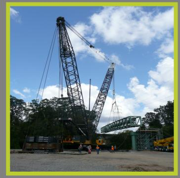
Lift under way. Notice the massive counterweight that was lifted only a few millimetres off the ground. The dogman on the far side of the river is visible.
