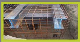
Pile cap prior to pouring of concrete.
