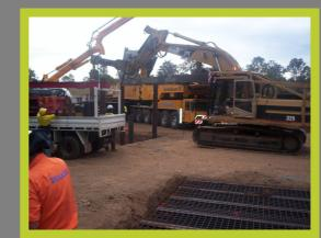
Installation of piles progress as other pile caps are prepared for concrete pouring.
