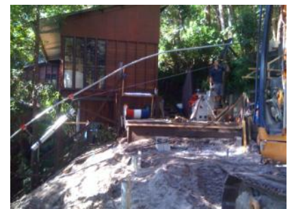
Flying fox carrying materials up the steep hill at Noosa
