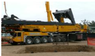
Crane ready to get in place
