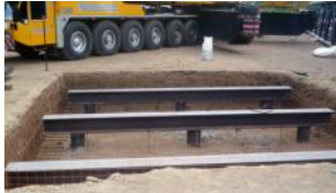
9 Piles Under Pile Cap
