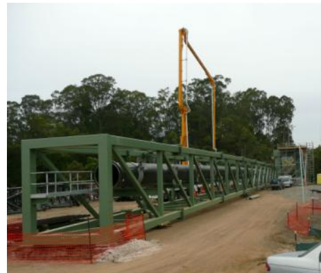
The Bridge Span to be Lifted
