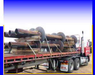
Transporting the Piles
