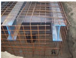
Closeup of Pile Cap
