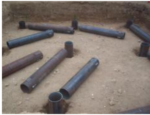
Getting the Piles ready
